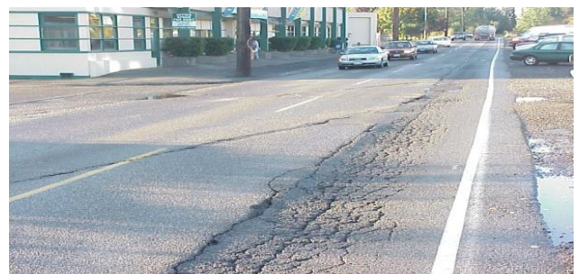
Fig1.1 Rutting phenomenon occurrence in bituminous pavement
